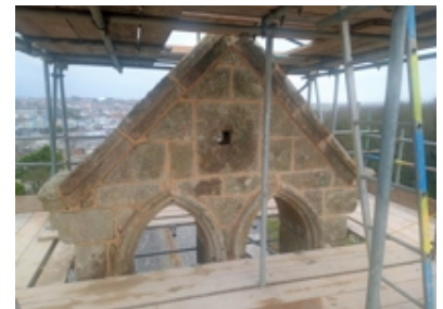
The newly repaired bellcote
